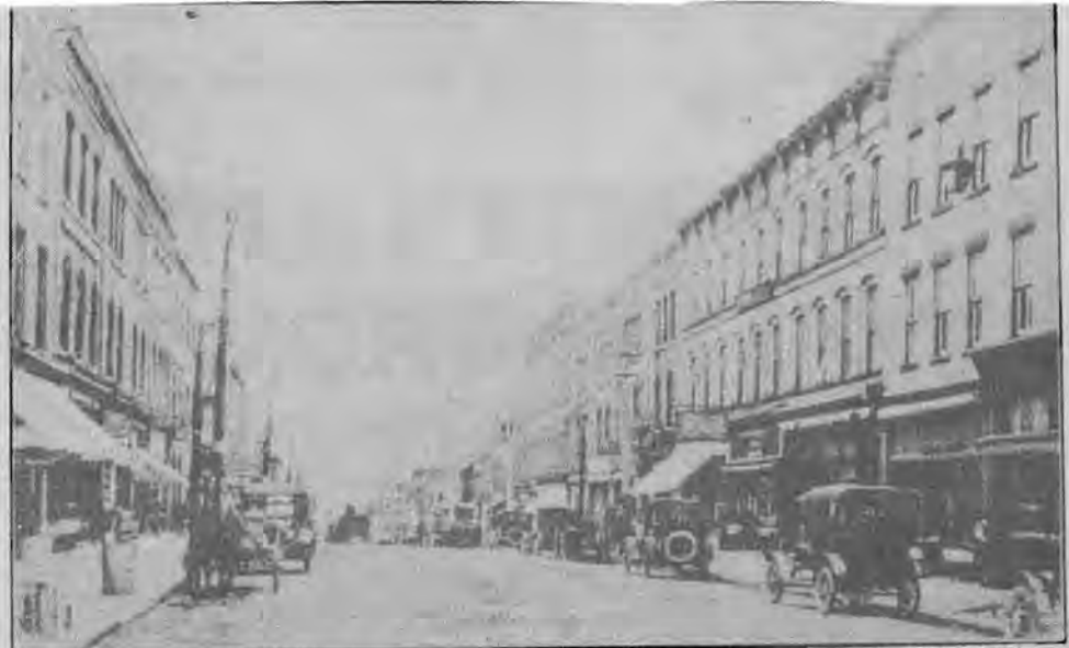
Horse driven buggies parked right beside the 'horseless carriages' that could be seen on Thames Street South in earlier days.
